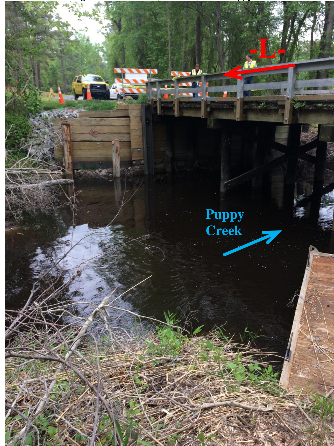
Bridge No. 61 on -L- (SR 1409) over Puppy Creek
